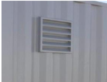
Figure 7: Non-descriptive example of fixed aluminium louver.
